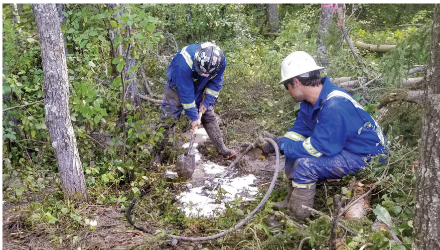
Cleanup crews flush forested impact site with Ivey-sol® surfactant.
