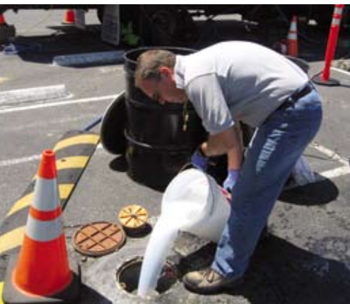
Ivey-sol is applied.
